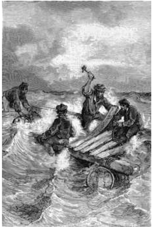
The work was begun
